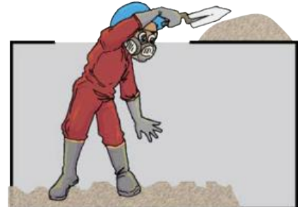
Removal of grit and settled sludge
